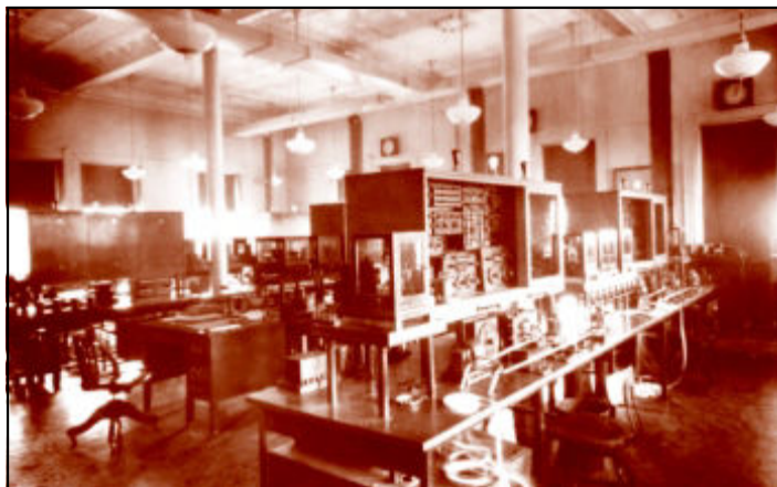
A typical Western Union “relay station” in the early 1900s. From here, received messages were retransmitted, or relayed, onto the proper destination circuit.
