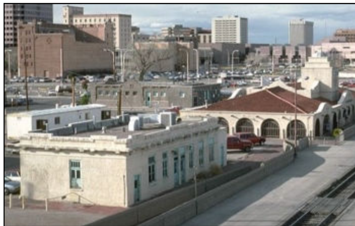
Photo by Even Werkema The Albuquerque Western Union Relay Station in 1991. The AT&SF depot on the right, with South-western design, was destroyed by fire two years later.
