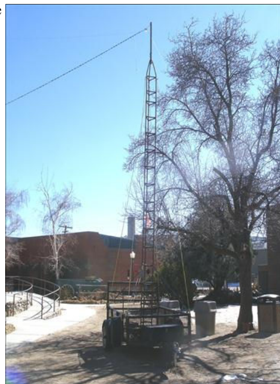
Pemberton Non-Stationary Antenna System (PNAS)
