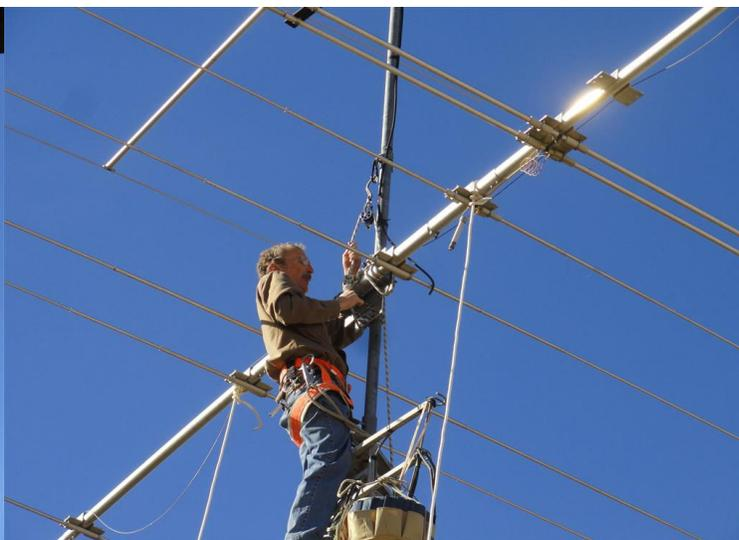
*Above -- Bud Semon, N7CW removing Dick's Force 12 C-31XR beam from his U.S. Tower*
