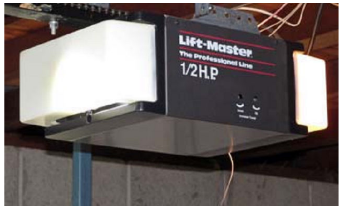
Garage door opener has built-in lampholders at each end. Wire antenna hangs down for reception of the 390 MHz remote control transmitter.
