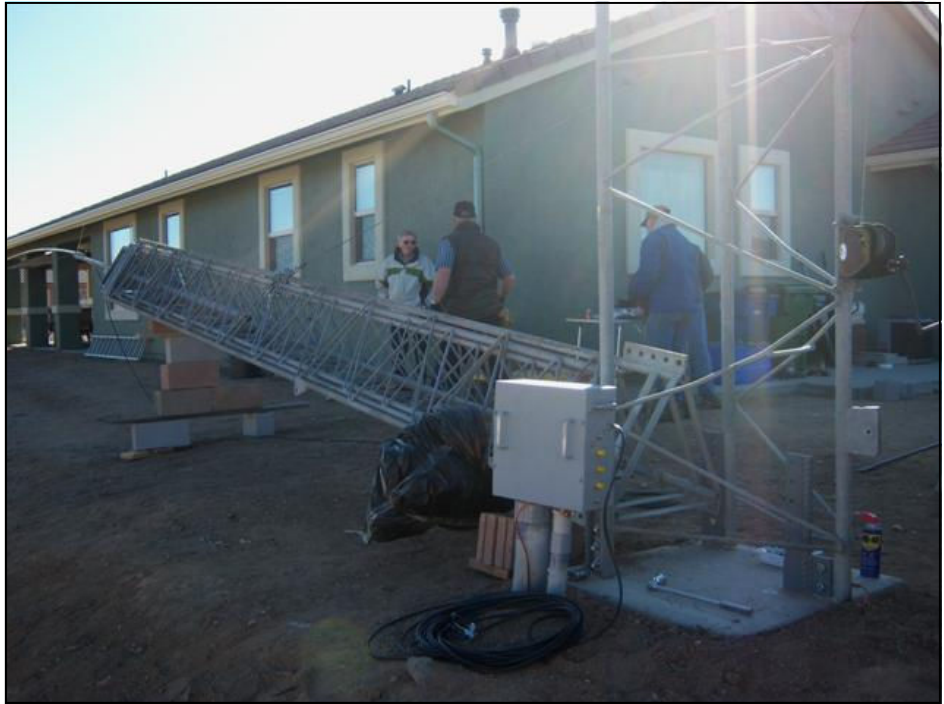
Tower mounted to base, ready to raise.
