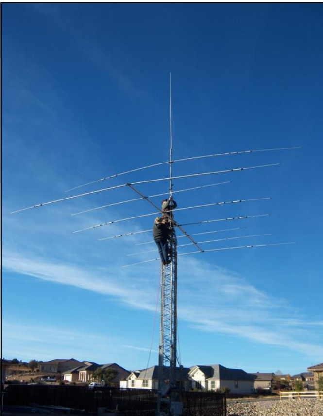
TH7 Yagi is attached to mast by Neil and Bob.
