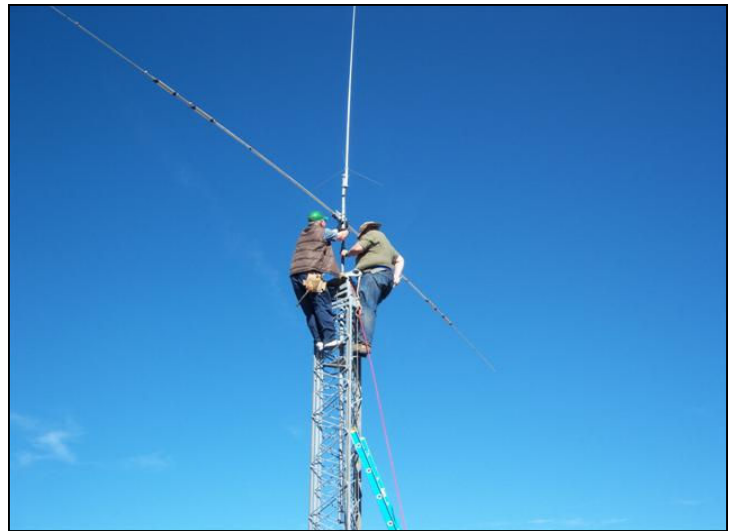
WARC rotatable dipole is attached to the mast by Neil, KA7JAS and Bob, KJ7SJ.
