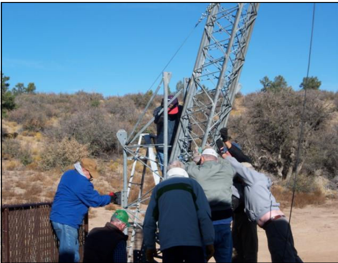
Tower almost fully upright. Tom, WN7E operating the hand winch.
