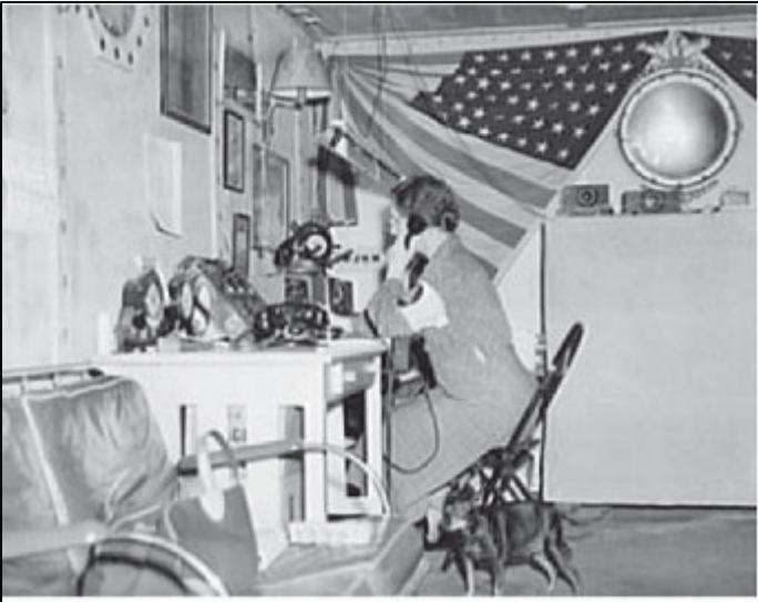
A War Emergency Radio Service transmitter-receiver keeps this air raid warden post in direct communication with the community Civilian Defense Control center. The set was constructed out of old home receivers by civilian radio volunteers. [Library of Congress picture.]
