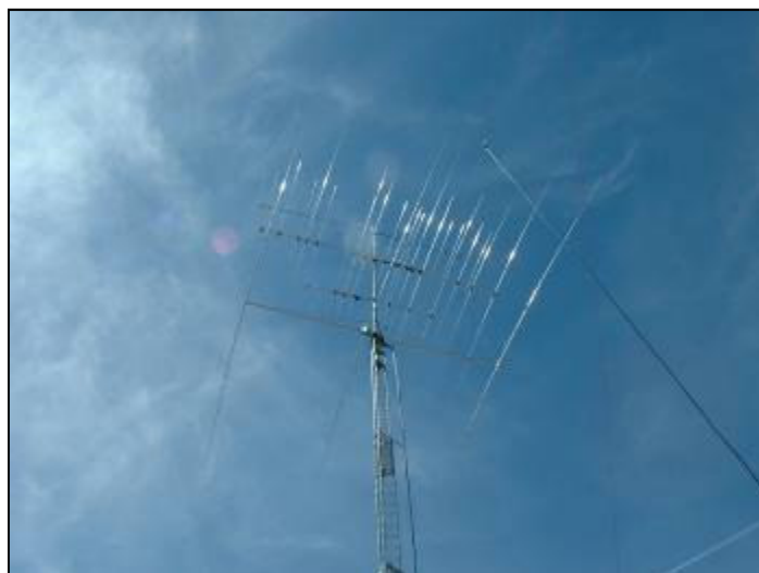
Bud's Yagis and Vertical stacked on a 90 Foot Heavy Duty Telescoping Tower
